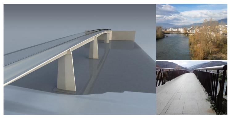
The structure of this pedestrian bridge consists of a deck with four spans of 20.00 + 25.00 + 48.50 + 21.50 m between axes with a total length of 115.00 m. The deck width is a constant 3.00 m.
